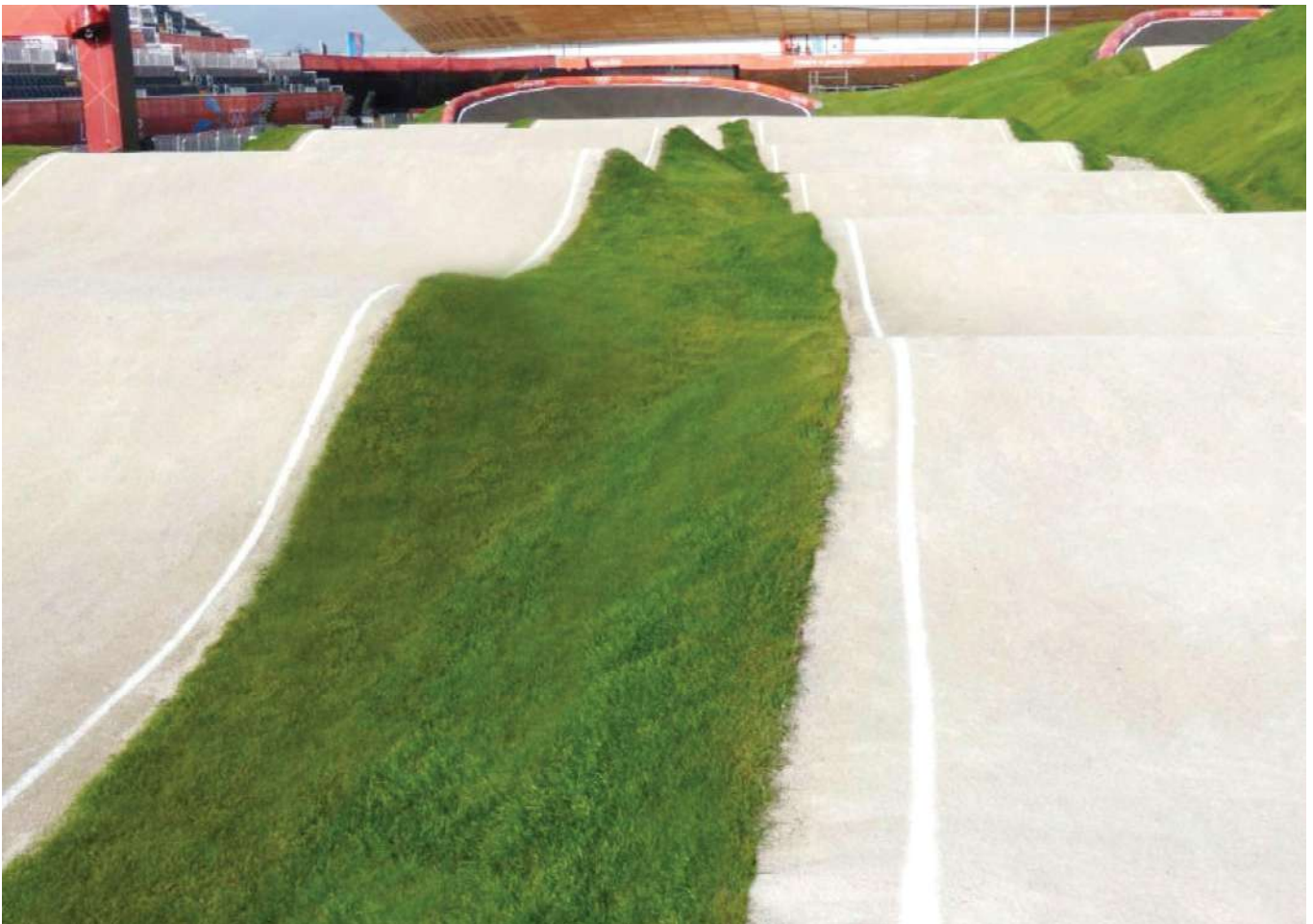
Straight 3 London 2012 olympic track (UK)
